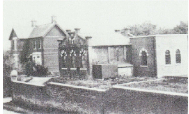
Figure 1. Haverhill Waterworks and Managers House, Burton End
