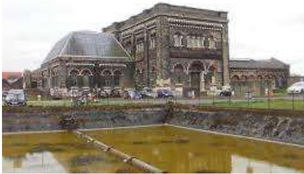
Figure 5. Crossness Pumping Station
